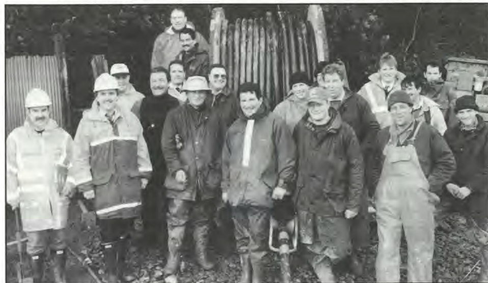
The cable laying team, comprising Manweb and BICC staff, and Duke of Edinburgh Award Scheme volunteers.
