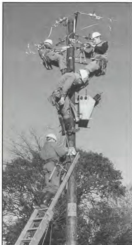
Manweb linesmen carry out repairs to the damaged overhead network.
